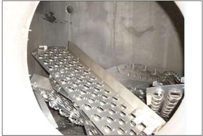
**Figure 2** - An internal photo confirming scan results and the trays had fallen down within the tower.
